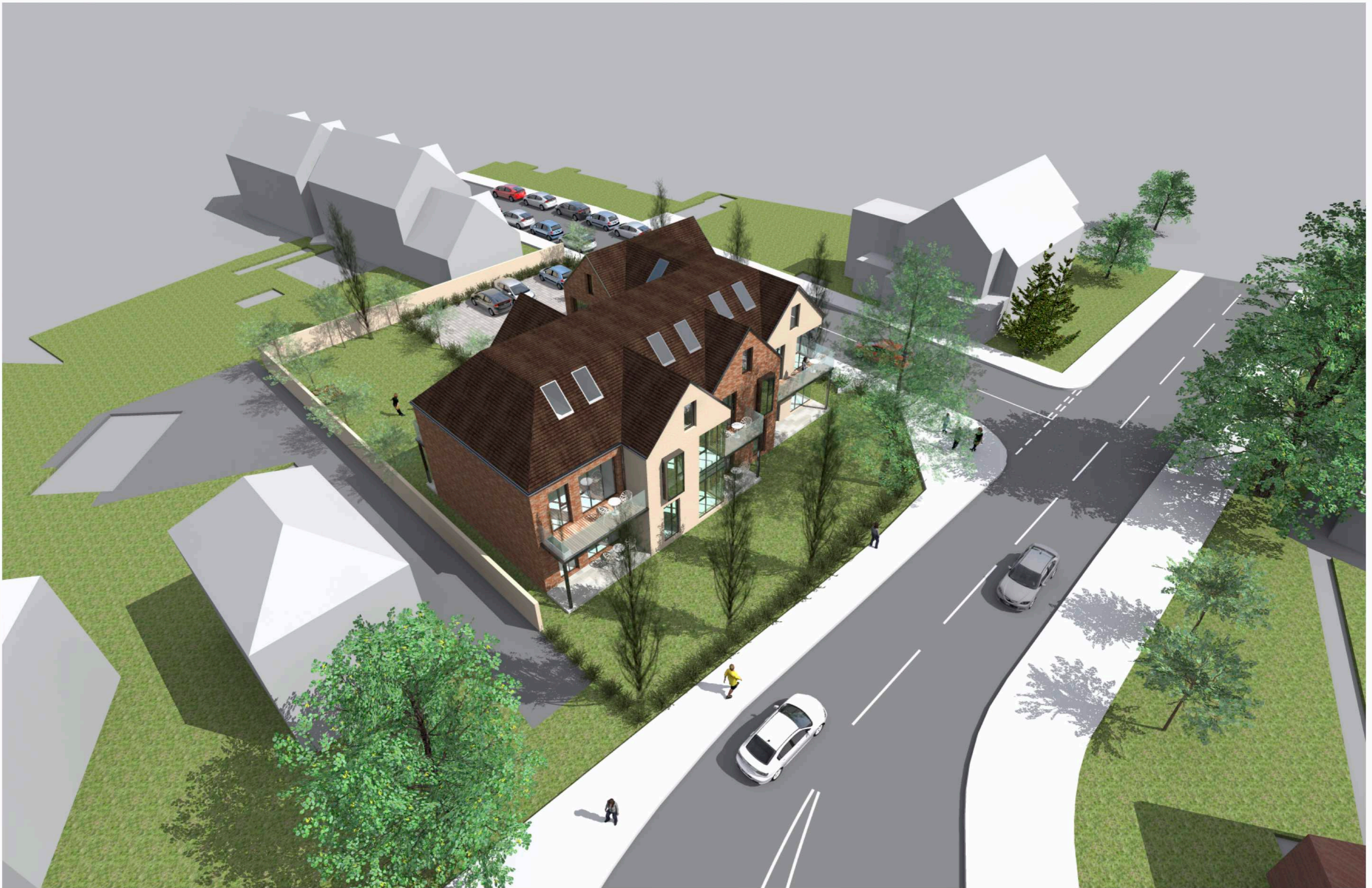
4. AERIAL VIEW FROM NORTH
